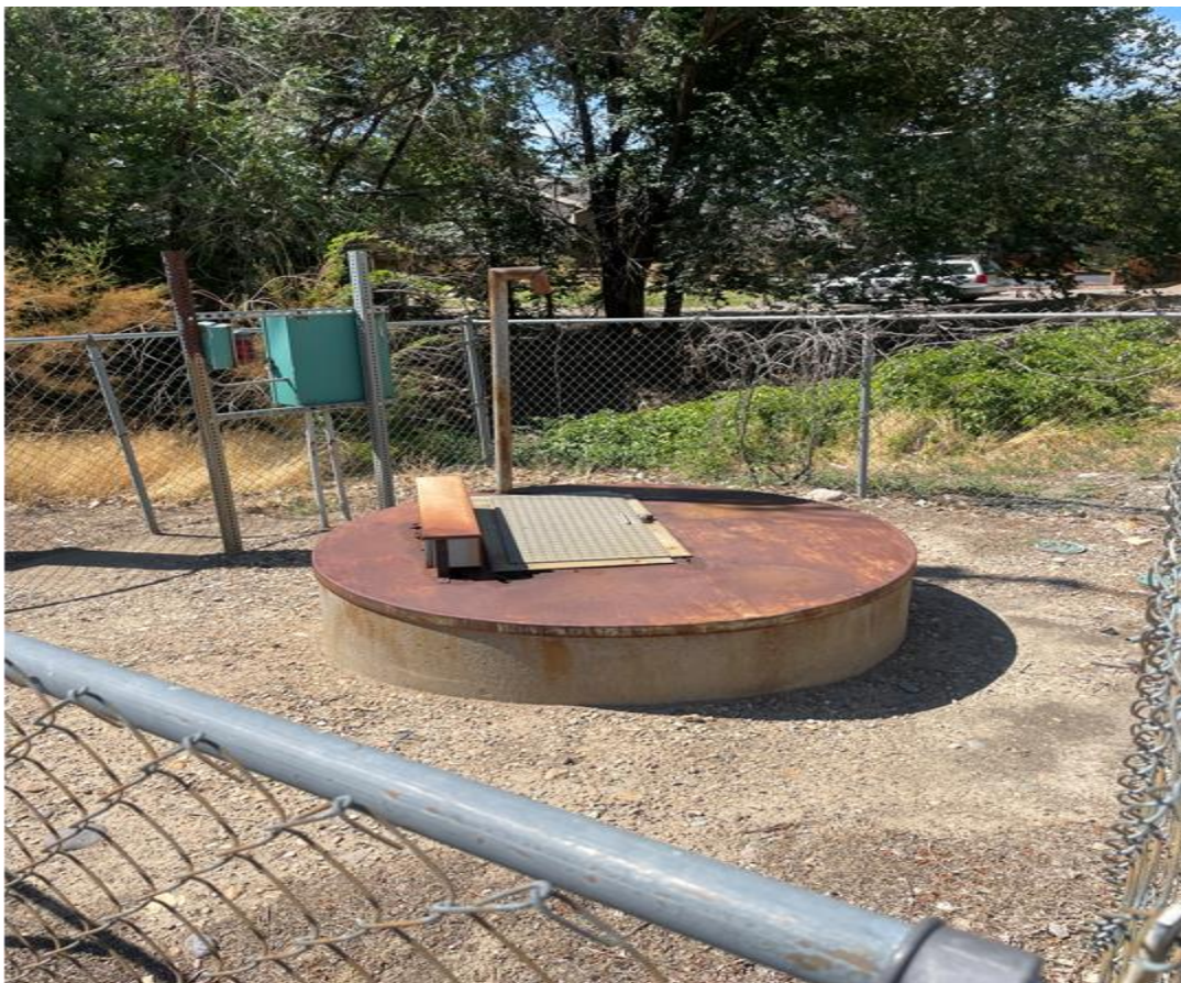
Troyer Lift Station with Drainage in background
