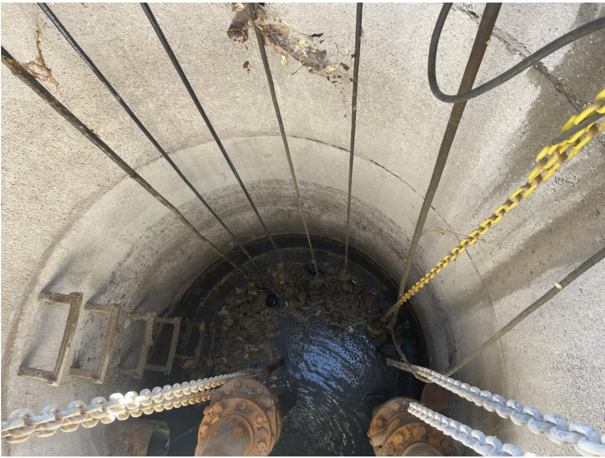
Vault for Troyer Lift Station
